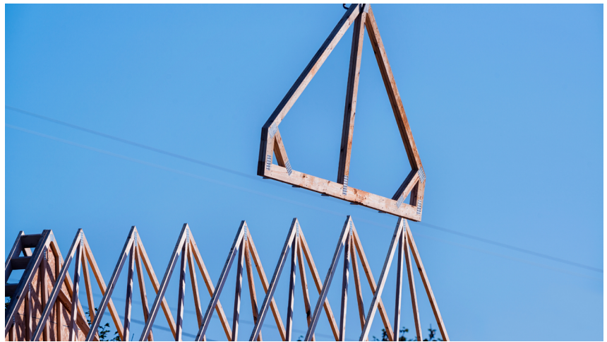
Wooden trusses installed to complete the roof structure.
