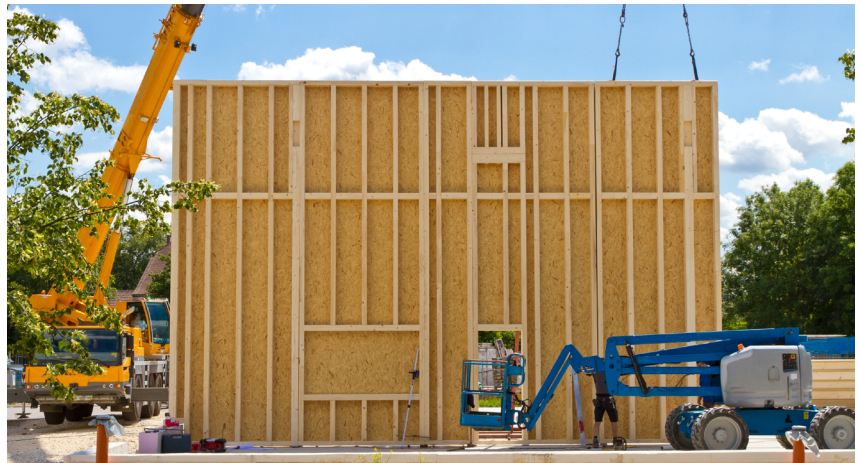
Prefabricated load-bearing wall featuring a wooden structure.
